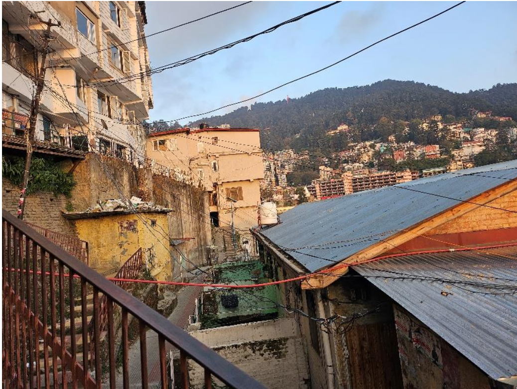
Figure 12: An area of Krishna Nagar, showing poorly planned construction, where one house sits right below another building on a hillside. Additionally, the lack of care with infrastructure can be seen through the proximity of electrical wiring to public pathways and homes (Author's own, 2023).
