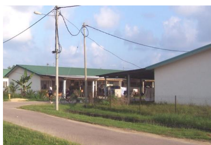
Single storey low-cost terraced
