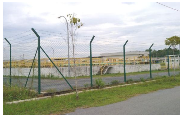
Centralised sewerage treatment plant
