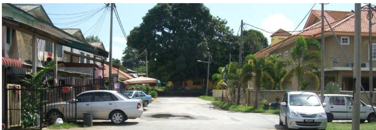
The low-cost housing component (left) is laid next to the commercial double storey terraced house (right) to promote social integration.
