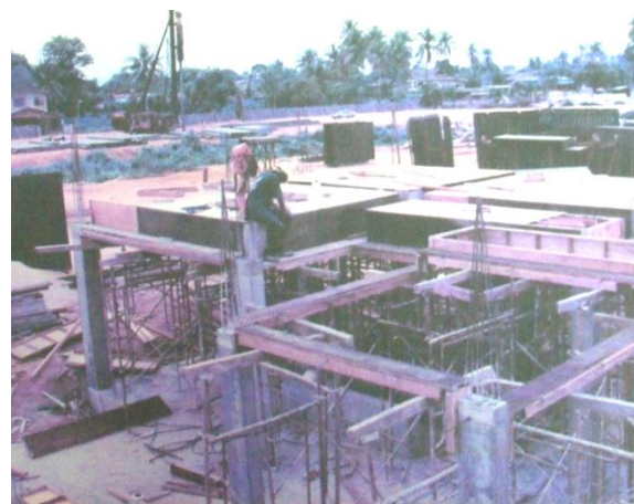
Current work on site
