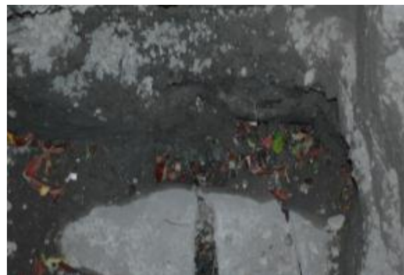
Figure 8.5: Manhole uplift, Dallington, 25 September 2010 (Source: Author's own)
