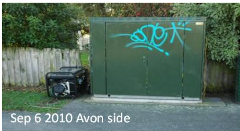
Photo 8.12: Application of portable power generator after the earthquake in WWPS (Source: Author's own)
