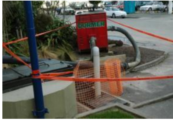
Figure 8.3: Discharge of wastewater directly to the river due to WWPS failure (Kaiapoi 24 September 2010) (Source: Author's own)
