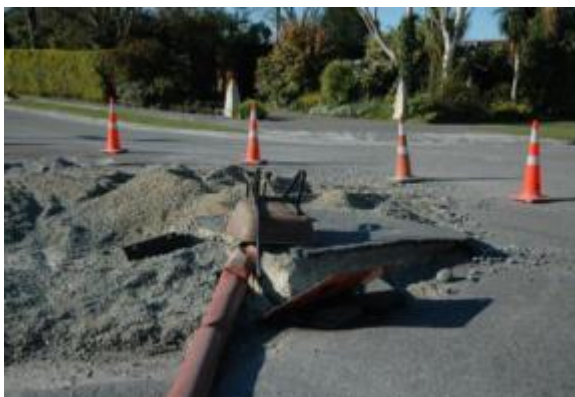
Figure 8.5: Manhole uplift, Dallington, 25 September 2010 (Source: Author's own)
