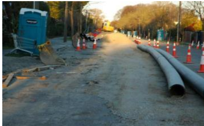
Photo 8.26: Replacement of the whole wastewater pipeline, Avonside 25 September 2010 (Source: Author's own)
