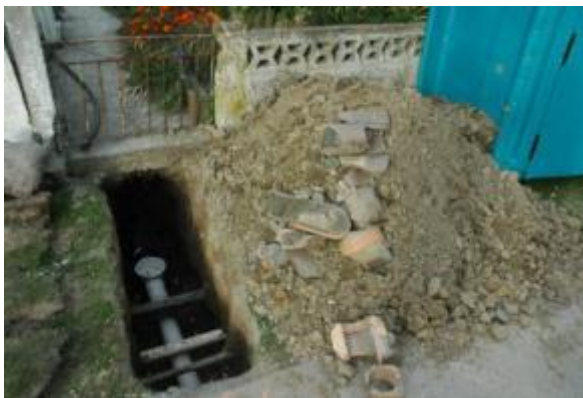
Figure 8.25: Residential building sanitary connection failures, Kaiapoi, 29 September 2010 (Source: Author's own)
