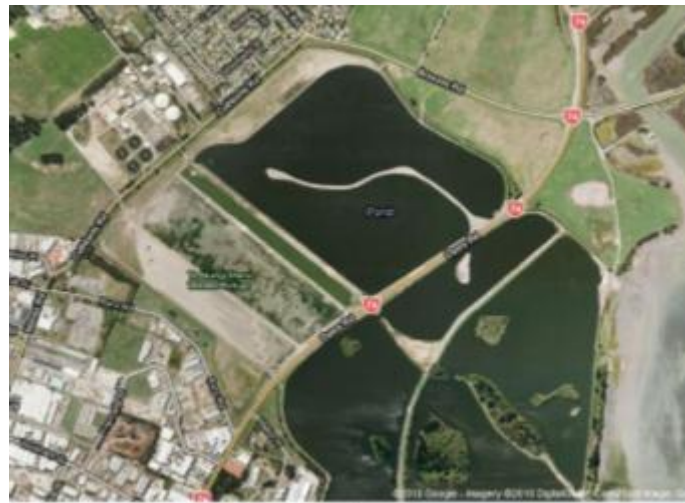
Figure 8.6: The main wastewater treatment plant in Bromley, Christchurch (Google Map 2010)
