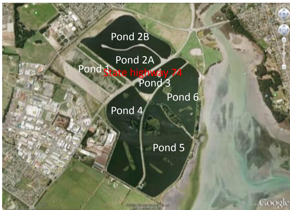
Figure 8.7: The Christchurch wastewater treatment plant ponds (Google map)
