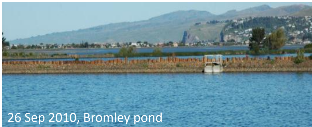
Photo 8.11: Sheet piles installed in the Christchurch wastewater system (Source: Author’s own)
