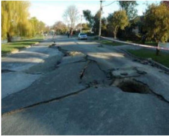
Figure 8.49: Inaccessible roads, 6 Sep. 2010 Christchurch (left severe road damage, right pipe breakages and debris) (Source: Author's own)
