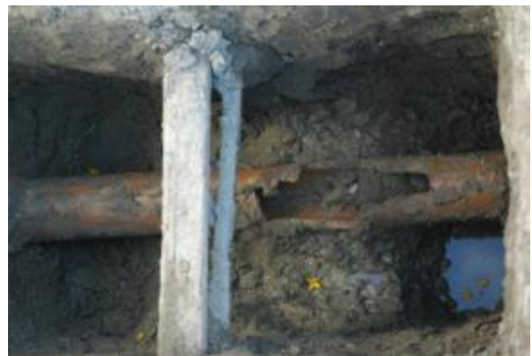
Figure 8.25: Residential building sanitary connection failures, Kaiapoi, 29 September 2010 (Source: Author's own)
