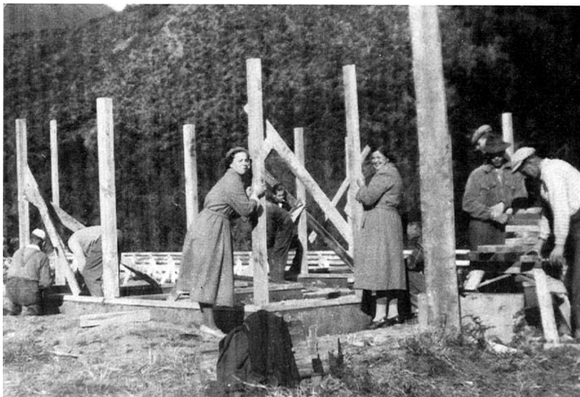
Figure 8 Men and Women Building the sauna in Kawerau in 1955 (Koivukangas, 1996, p. 215)
