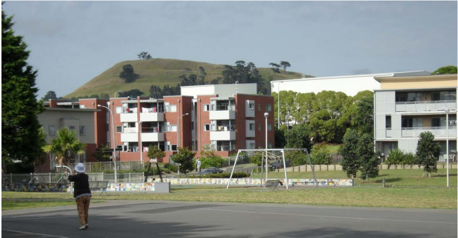
Figure 2: Talbot Park after renewal project
