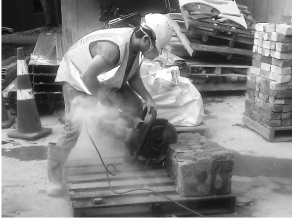
(a) cutting of extracted URM section
