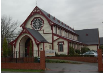
(a) timber church of St Andrews, Merivale, 1857
