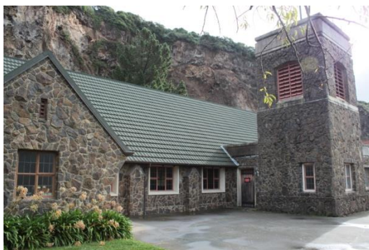
Figure 14 – Example of an undamaged church classified red due to instability of the slope shown in the background (All Saints, stone, Sumner).
