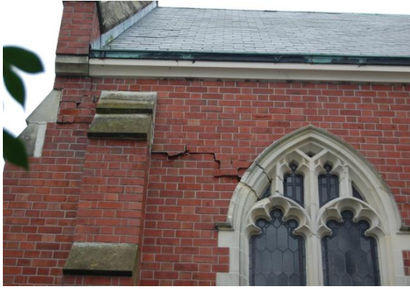
(a) shear damage in the longitudinal walls (mechanism 6), outside (Nazareth's House church, brick, Sydenham)
