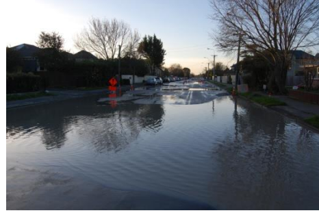
(b) liquefaction in the Christchurch City centre
