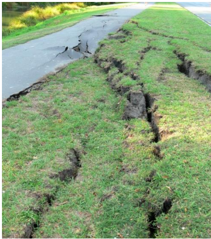
(c) lateral spreading along the Avon River
