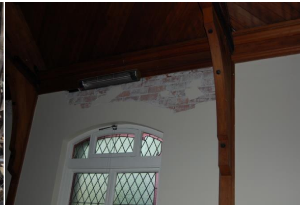
(d) hammering of the roof (mechanism 19), inside (Shirley Methodist, brick, Shirley)
