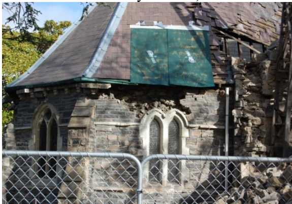
(a) shear damage in the longitudinal walls (mechanism 6), outside (Nazareth's House church, brick, Sydenham)
