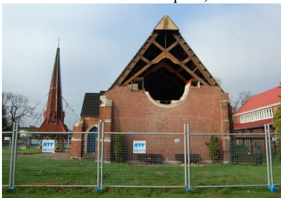
(c) hammering of the roof (mechanism 19), outside (St. John's, stone, Latimer Square)
