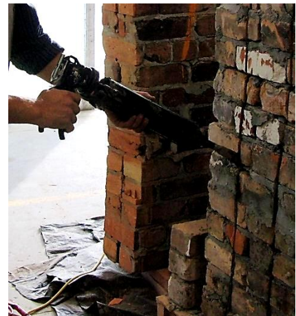
(c) grout injection
