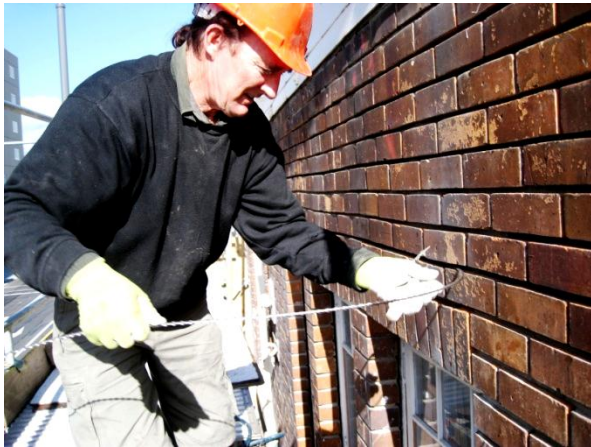
(c) bed joint insertion of TS bars
