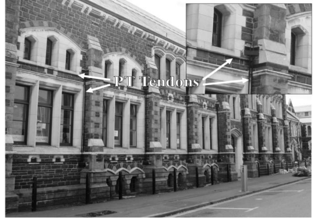
(b) external posttensioning
