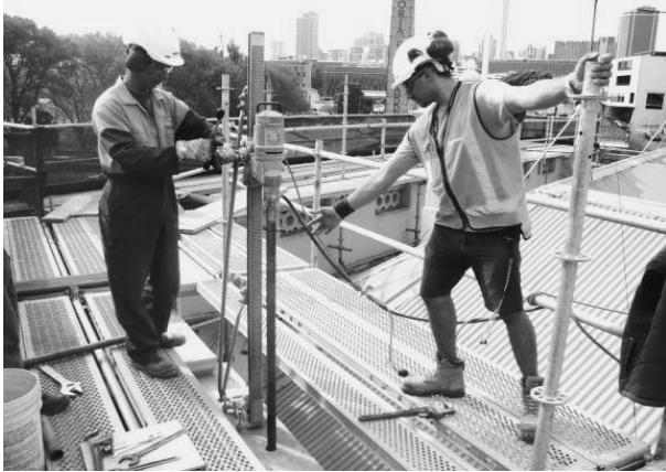
(a) coring operation for internal posttensioning
