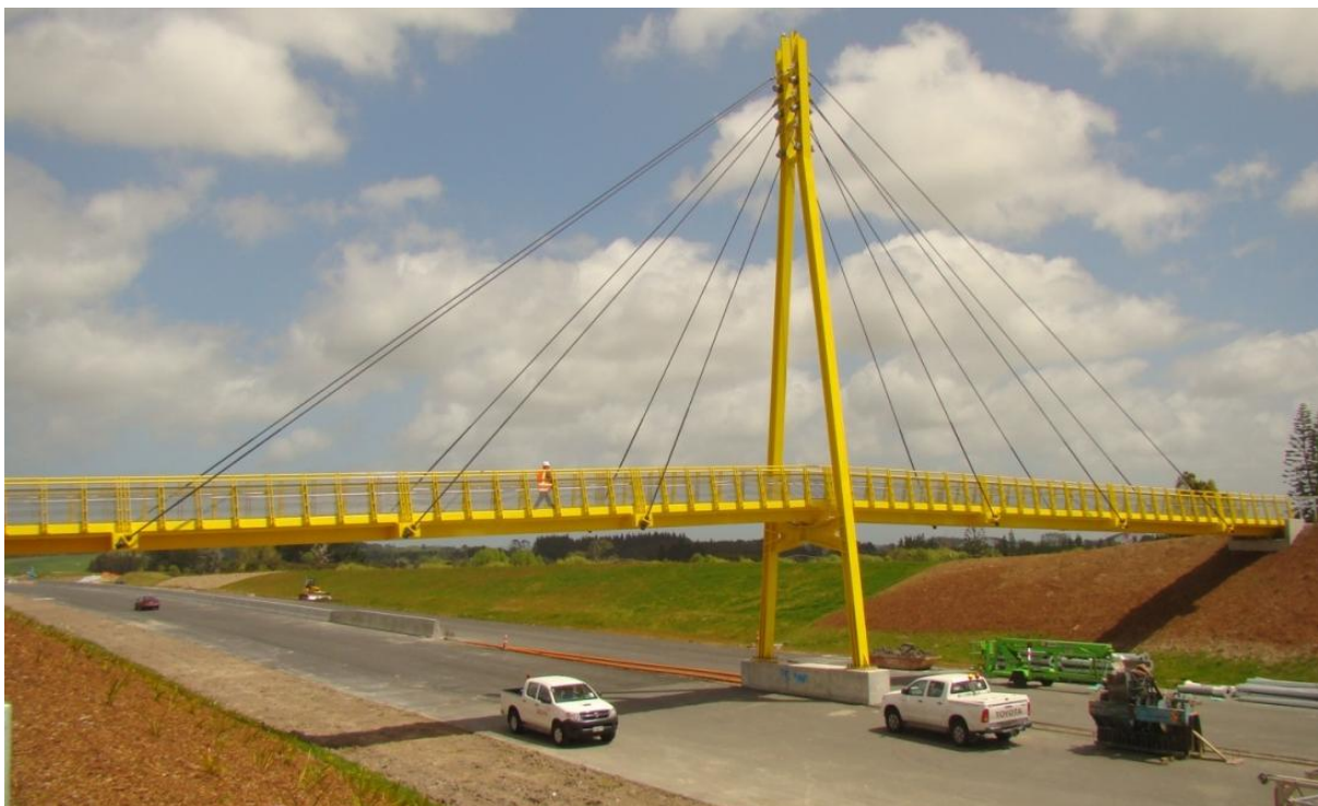
Figure 5.1. Full-scale cable-stayed footbridge.
