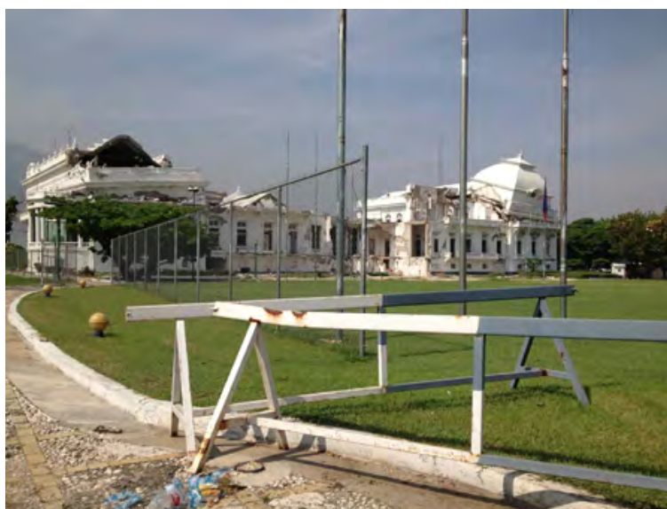
Figure 3-7: Haiti's National Government Palace after the 2010 earthquake
