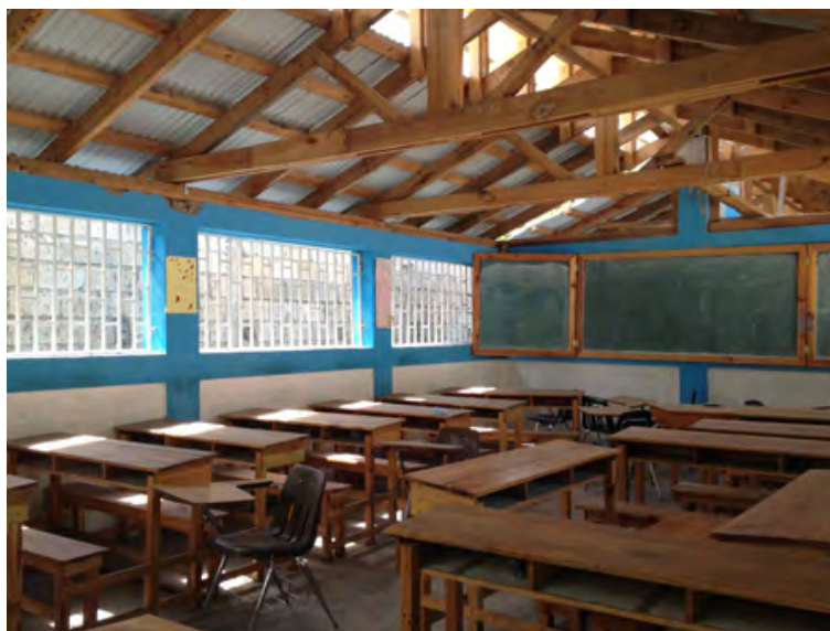
Figure 5-3: A classroom construction project for UNESCO by AFH Haiti
