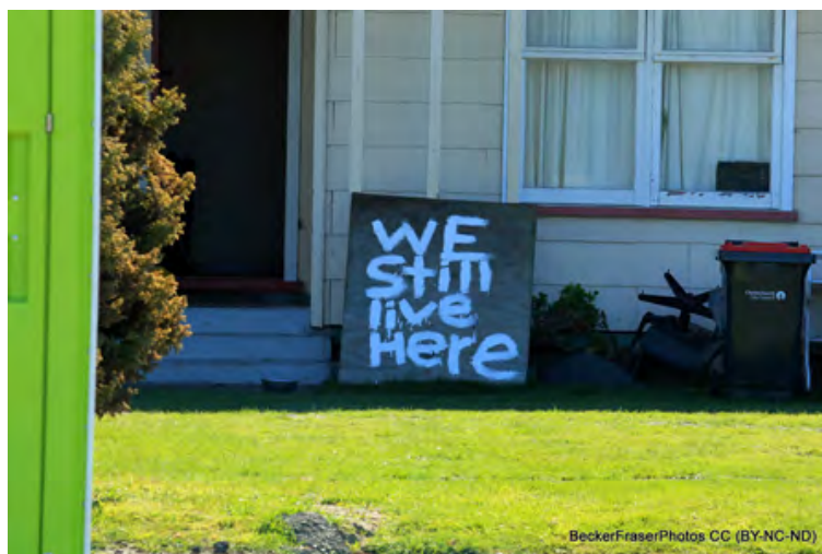
Figure 7-6: Becker, Ross (2011) Locksley Avenue. [photograph] Retrieved on 16 Aug 2013 from Picasa commons: https://picasaweb.google.com/114788127440201076357/EastChristchurch?noredirect=1#5725261347424036242 Copyright 2013 by RossFraserPhotos. Reprinted with permission.
