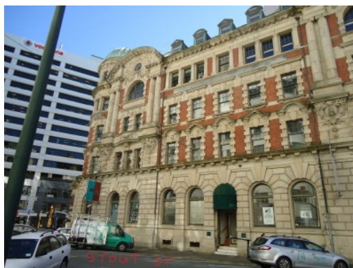
(a) Old Public Trust Building
