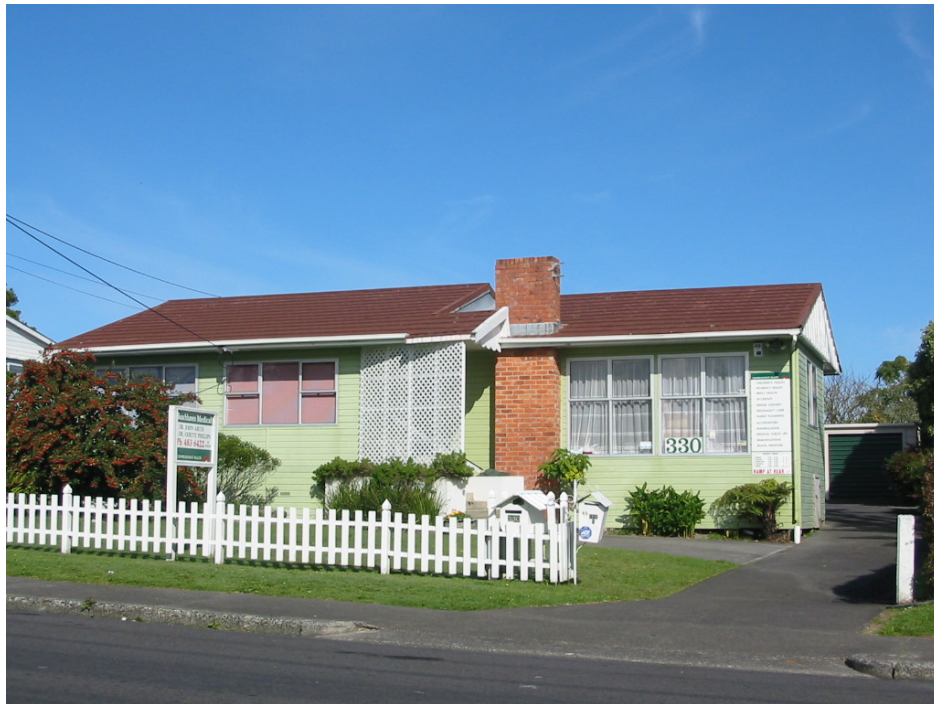
Figure 4.4 Auckland PHO GP Clinic (operated out of a converted dwelling), 2007.
