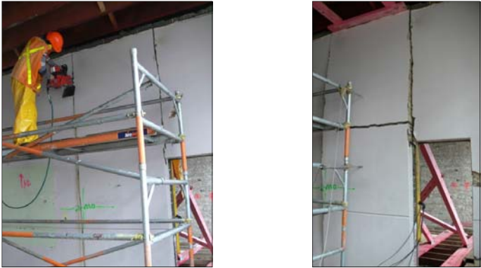
(a) Cutting through concrete ring beam (b) AS-SS test crack location
