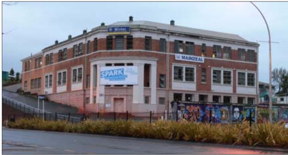
(c) Wintec Block F, located at the intersection of Anglesea and Ward Streets, Hamilton
