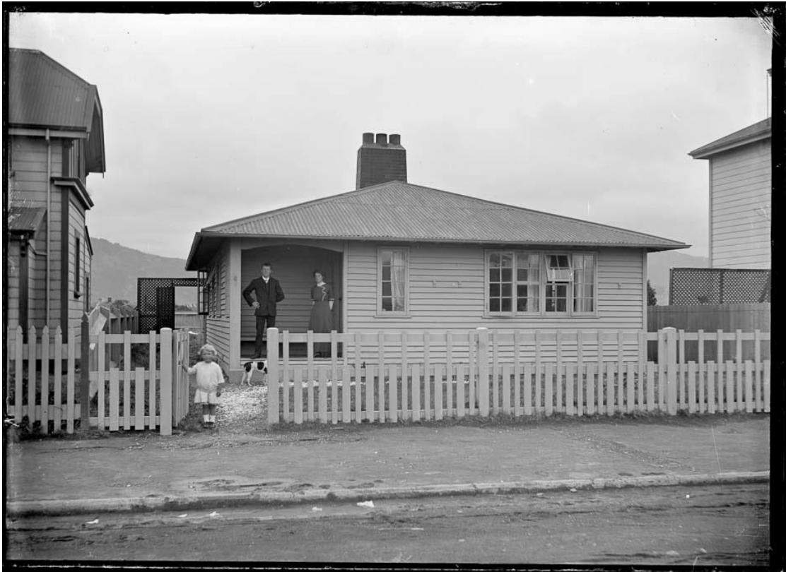
Figure 3.1: First worker's house in Petone 1910 designed for married workers with children (Ministry of Culture and Heritage, 2014).
