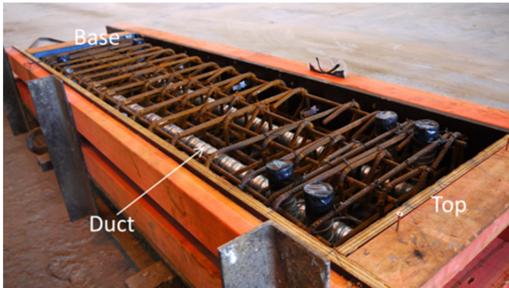
(a) Vertical ducts for PT bars
