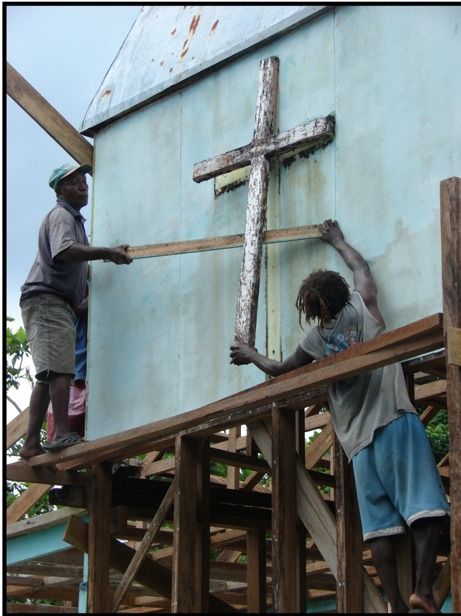
Figure 4 – Members of the Methodist Church disassemble the damaged church building
