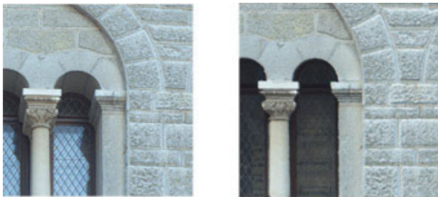
Figure 12: Left: original panorama image, right: processed ortho image.
