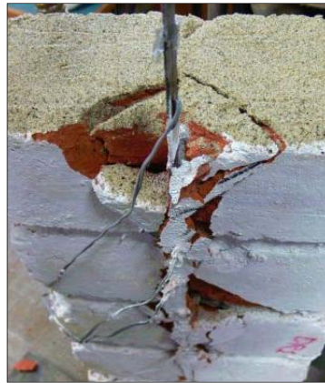
(b) Top view of prism following failure B1-4-15-(6/20)
