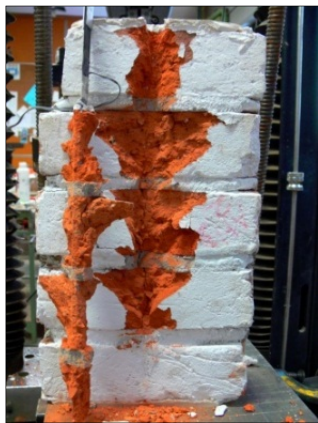
Brick surface CFRP strip Epoxy Failure plane (a) Trapezoidal failure plane, H F2-4-15-(6/20)
