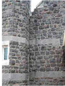
(b) St. Mary's Anglican Church: detachment of the bell tower from the nave
