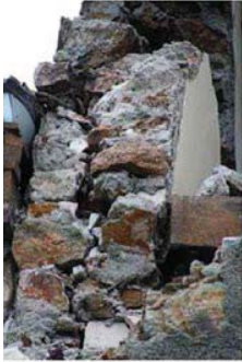
(a) Time Ball Station with multiple-leaf stone masonry
