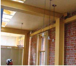
(c) Laurie and Wilsons Auctioneers building. Presence of steel frame
