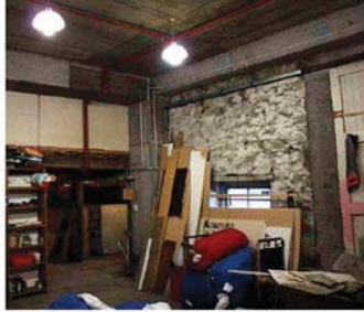
(d) Former Malthouse Building. Presence of reinforced concrete frame
