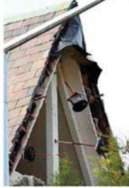
(a) Cramner Court. Gable ended out-of-plane wall failure.
