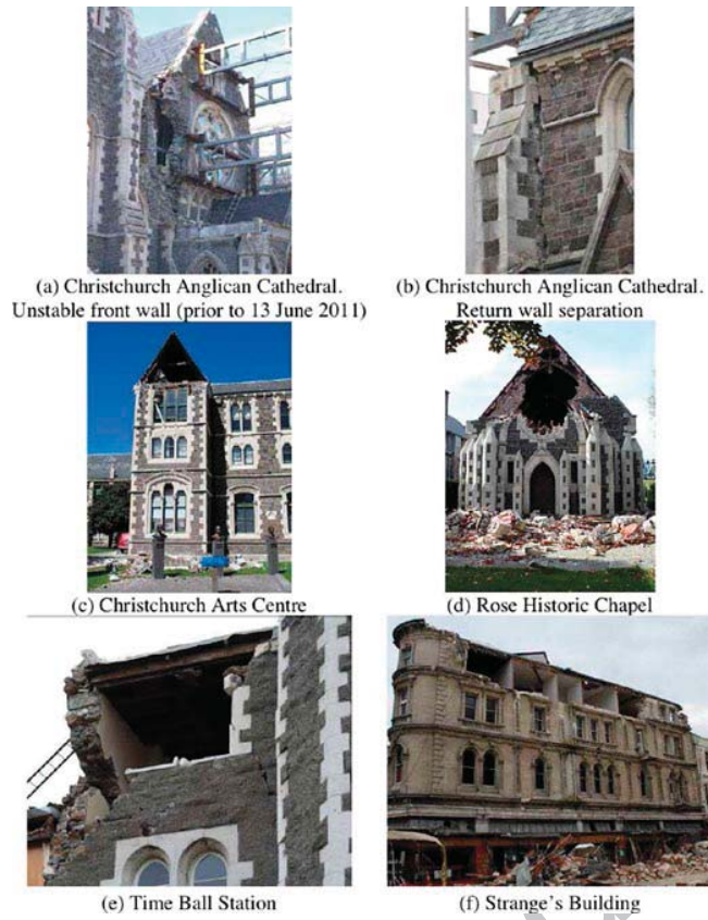
Figure 15. Examples of global and local out-of-plane overturning mechanisms of façades
