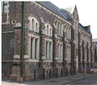
(e) Former Chemistry Department, Christchurch Arts Centre. Use of post-tensioning.
