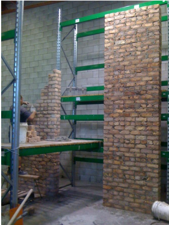
Figure 1: Construction of clay brick unreinforced masonry walls
