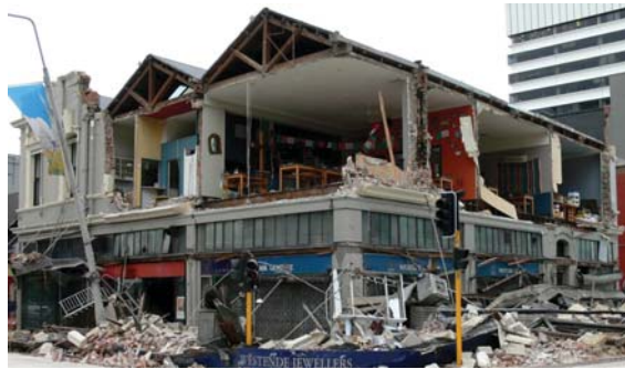
FIG. 14: Out-of-plane wall failure, Christchurch 2011 (credit: D. Dizhur)
