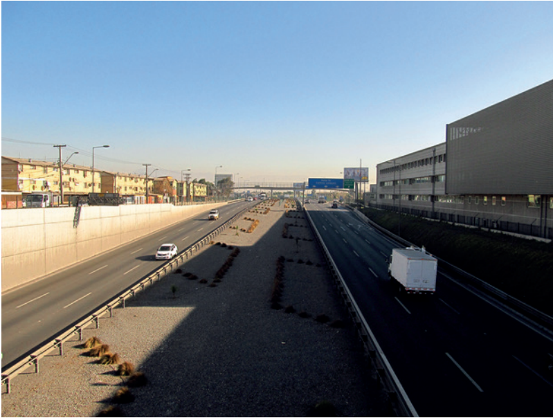
Figure 2.4. The interstitial boundary space between Lo Espejo and Pedro Aguirre Cerda communes (author's photo, May 2014)
