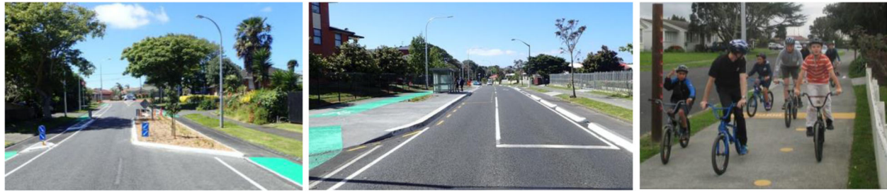
Fig. 3 Examples of intervention infrastructure. A demonstrates physically separated cycleways, road narrowing and indigenous planting on a local street previously being used like an arterial road. B demonstrates physically separated cycleways, widened and smoothed footpaths and treatment of cycleways around a bus stop, on an arterial road. C shows a greatly widened and smoothed shared footpath/cycle nursery, along with indigenous markings (marker posts and paintwork) on a local street, as part of a fitness circuit (Photograph credits: Richard Scott, Mackie Research 2017 and Stuart Houghton, Boffa Miskell 2017, with permission)
