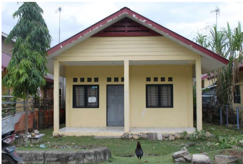
Figure 4.3. House provided by Australian Red Cross in Labuy
