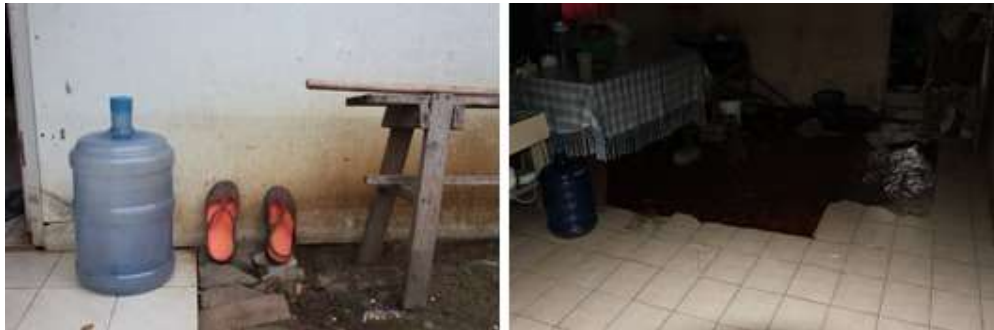
Figure 4.14. Level of inundating water in a flooded house
