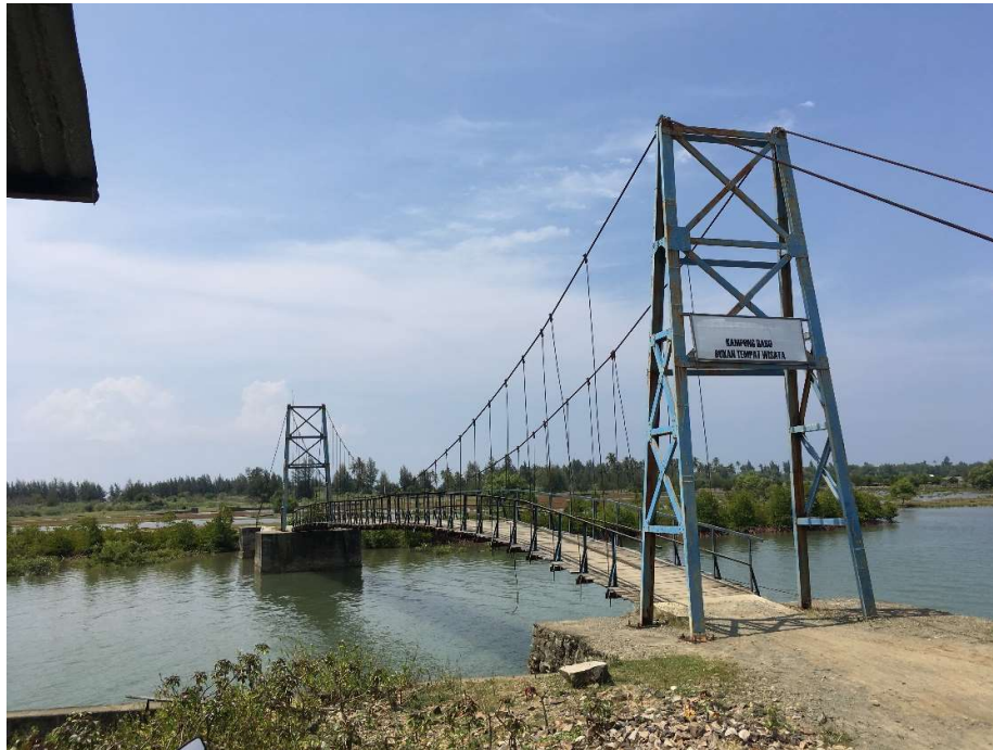
Figure 4.10. Pedestrian suspension bridge to the old Gampong Baru
