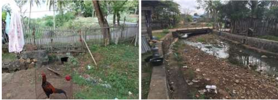
Figure 4.15. Poor drainage in Budha Tzu Chi Neuhuen
