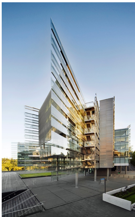
Figure. 1. Owen G. Glenn Building at the University of Auckland
