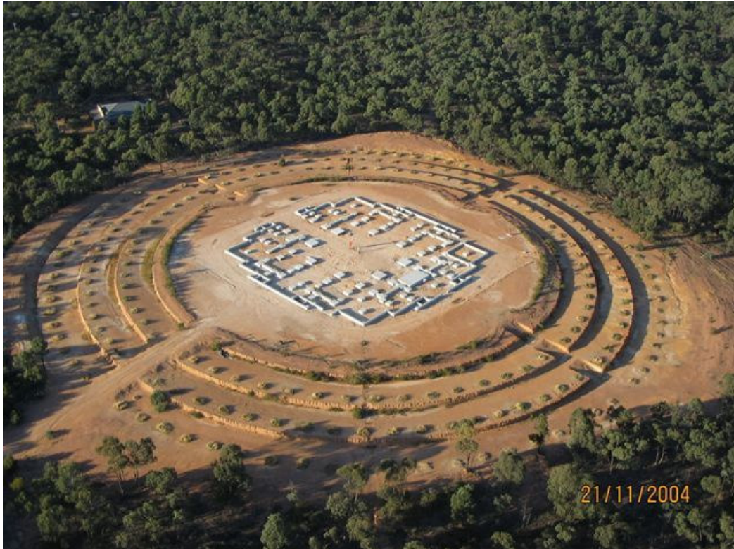
Aerial photo of stupa foundations, courtesy of Wayne Maconachie
