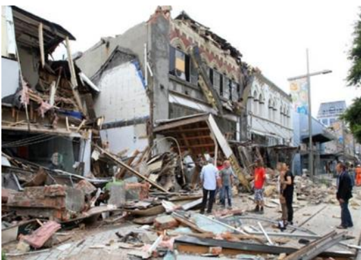
Figure 1.1: City Mall after 22 February earthquake 2011
