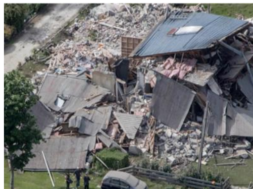
Figure 1.2: Kaikoura earthquake 14 of November
