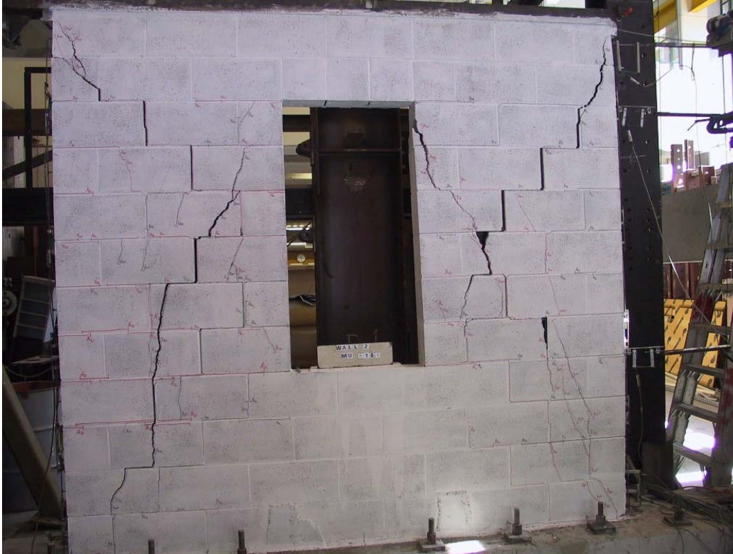
Figure 6.21 Series B, condition of Wall B2 at end of testing.
