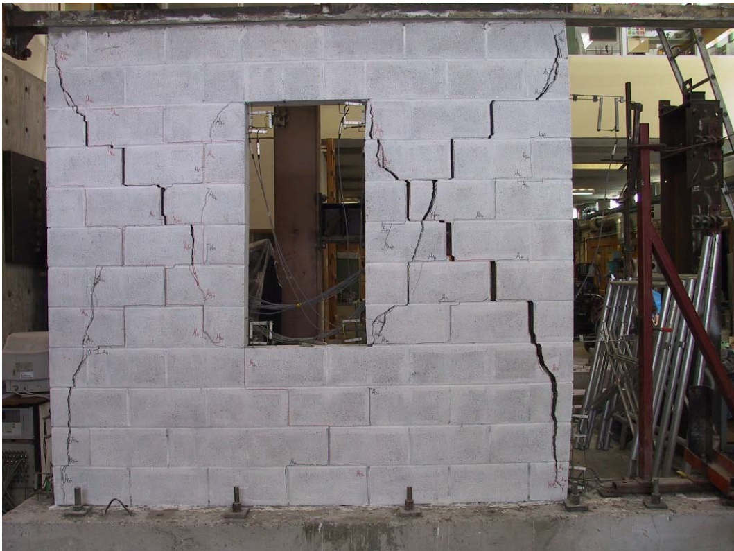
Figure 6.22 Series B, condition of Wall B4 at end of testing.
