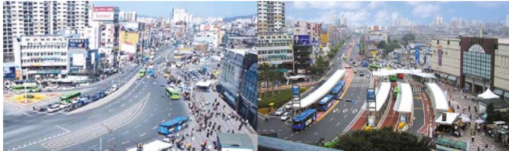
Figure 25 - Cheongnyangi bus and train interchange before (left) and after (right) the BRT project
