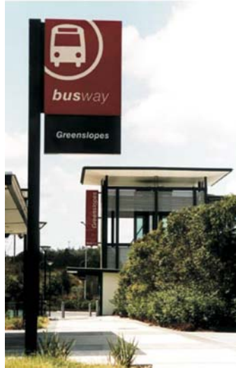
Figure 6 - Utilisation of consistent signage visual design and stations' architectural design on Brisbane BRT
