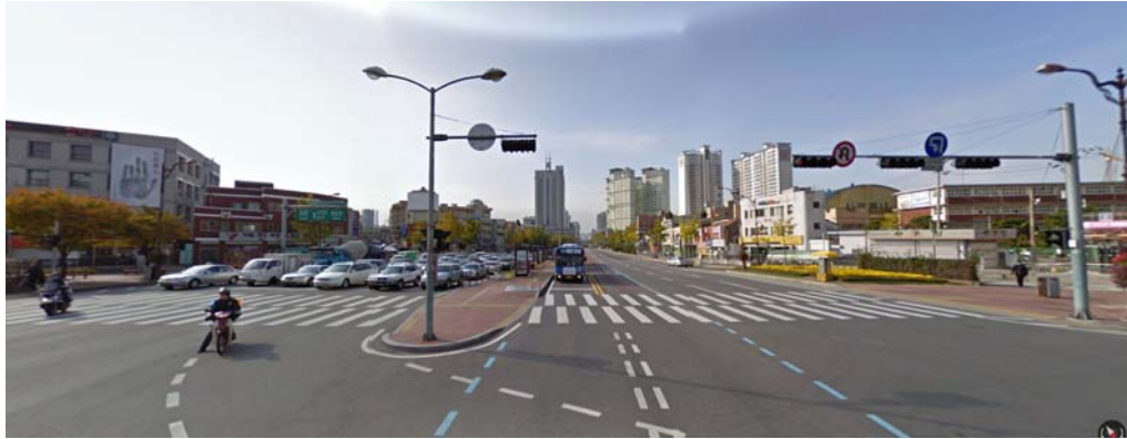
Figure 23 - Seoul BRT median lanes at Hangang Avenue-Baekbeom Road intersection
