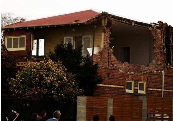
Figure 10. Examples of out-of-plane failures in cavity walls.
