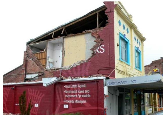
Figure 10. Examples of out-of-plane failures in cavity walls.
