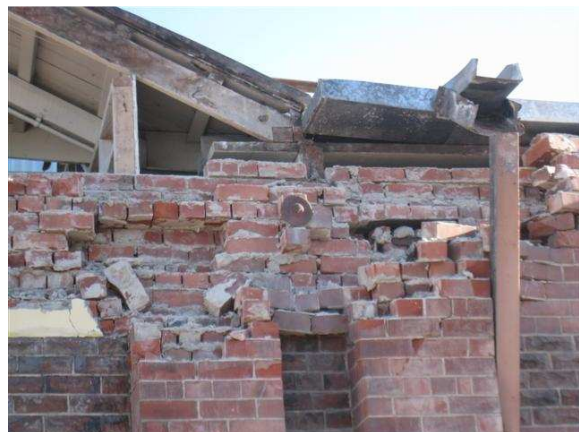
(b) Wall anchor still intact
