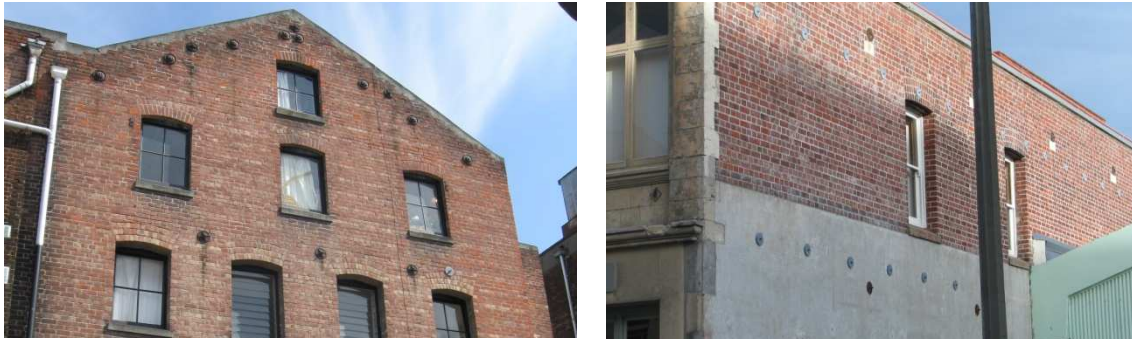
Figure 16. Successful wall-floor and wall-roof diaphragm anchorages.
