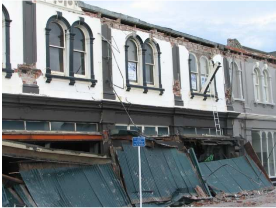
(a) Multiple front wall parapet failures
