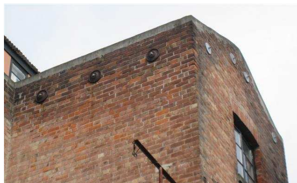
Figure 15. Successful gable end wall and side wall anchorages.
