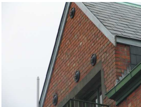
Figure 15. Successful gable end wall and side wall anchorages.
