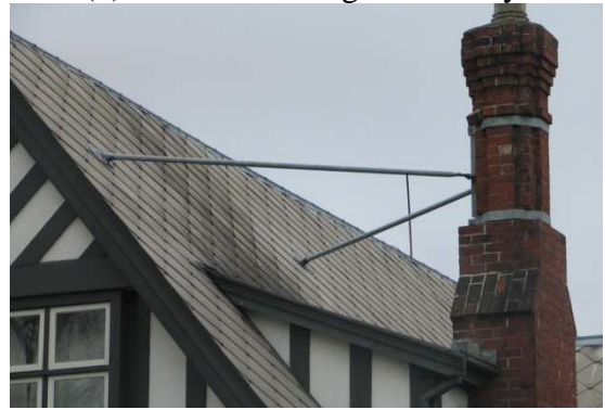
(d) Braced chimney performed well
