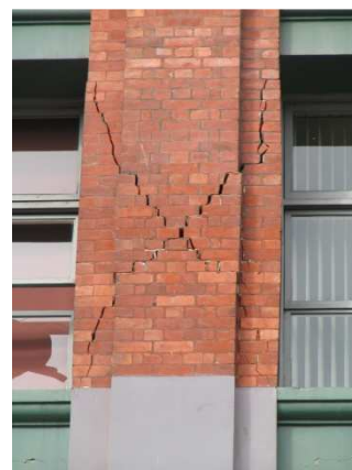
(b) North wall pier, level 3.
