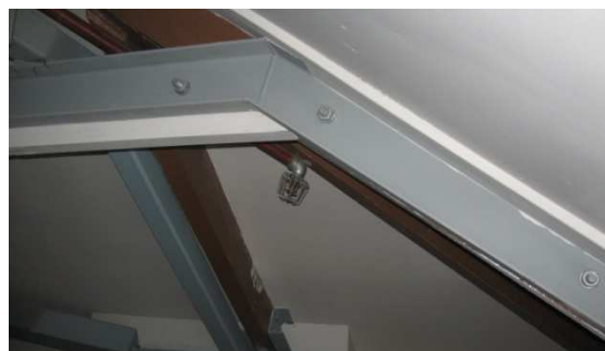
Figure 19 – Steel frame in roof
