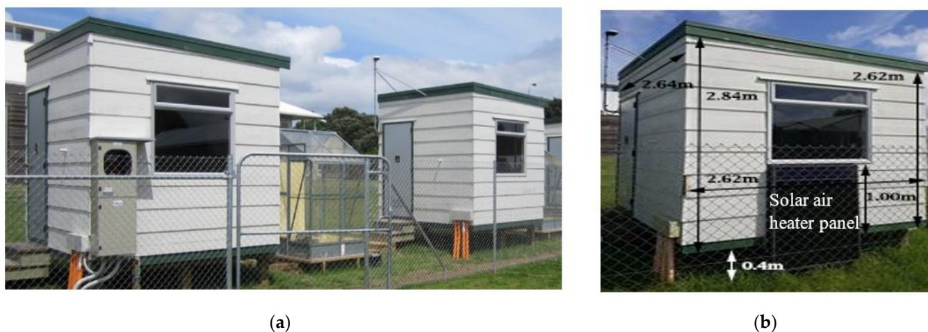
Figure 1. (a) The experimental test and control huts, located at the University of Auckland [22]. (b) The hut was supplied with a solar air heater panel [19].
