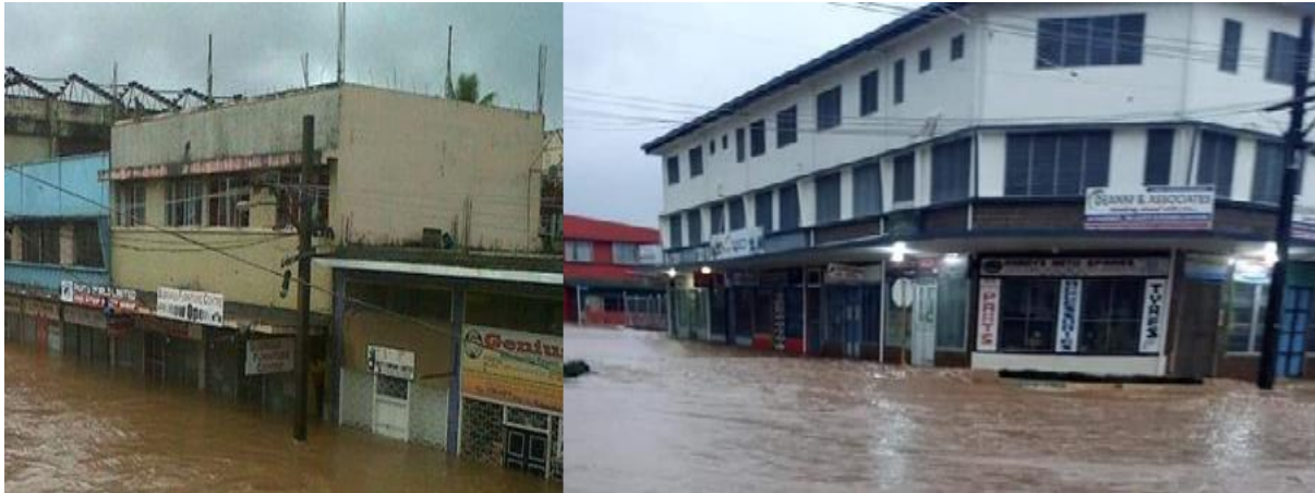
Figure 4.8: Ba town under water during April 2018 floods (Left image: water levels up to 4 feet. Right image: water levels up to 1.7 feet in height during the April 2018 floods) (Source, Sivendra Michael, Fieldwork, 2018).
