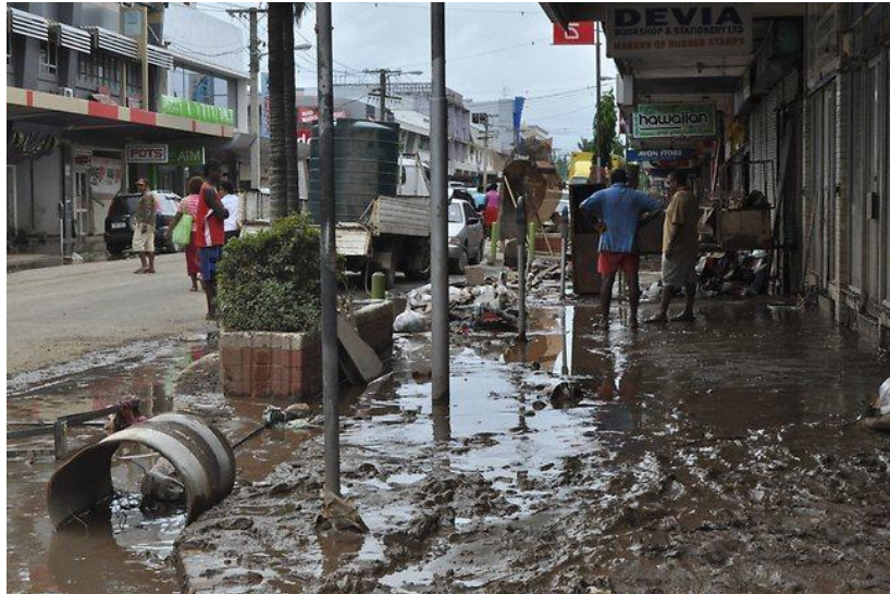
Figure 5.3 Damage from April 2018 floods (Source: Research participant, 2018 – consent obtained for using photograph)
