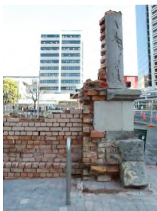
Fig. 3. Evtotia Photography (June 2016). Kaiapoi Fragment prior to dismantling and storage [Photograph, Reverb Consultancy Report]
