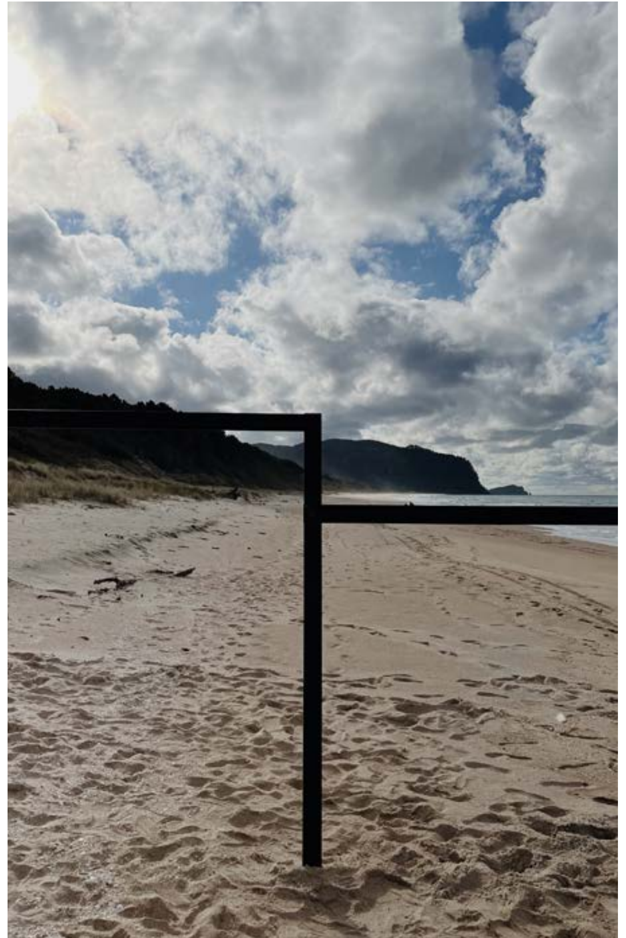
Figure 6: Image of a connection in the Opoutere Installation.
