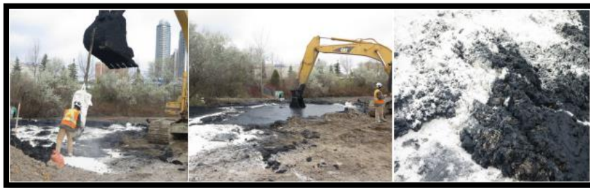
Figure 2-1: SAP Powder Applied to Wet Sediment (TRCA & CH2M Ltd, 2016)
