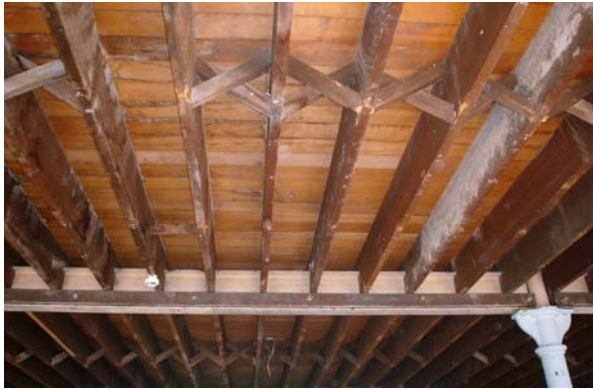
(a) Underside showing joists, sheathing and cross-bracing
