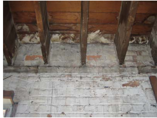
(b) Joists pocketed into URM perimeter wall
