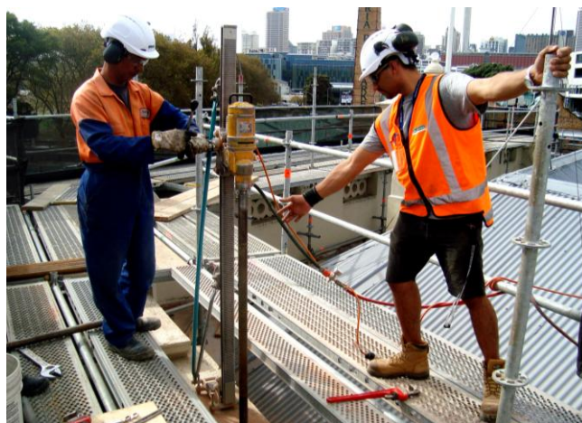
Figure 1. Coring Operation
