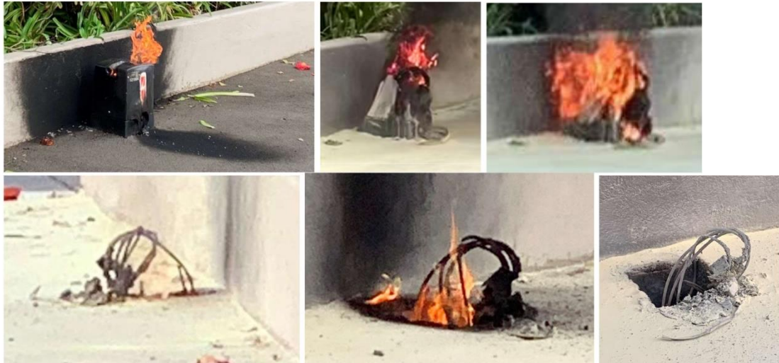
Figure 2 LV Pillar Fire Progression Over 90 Minutes [1]
